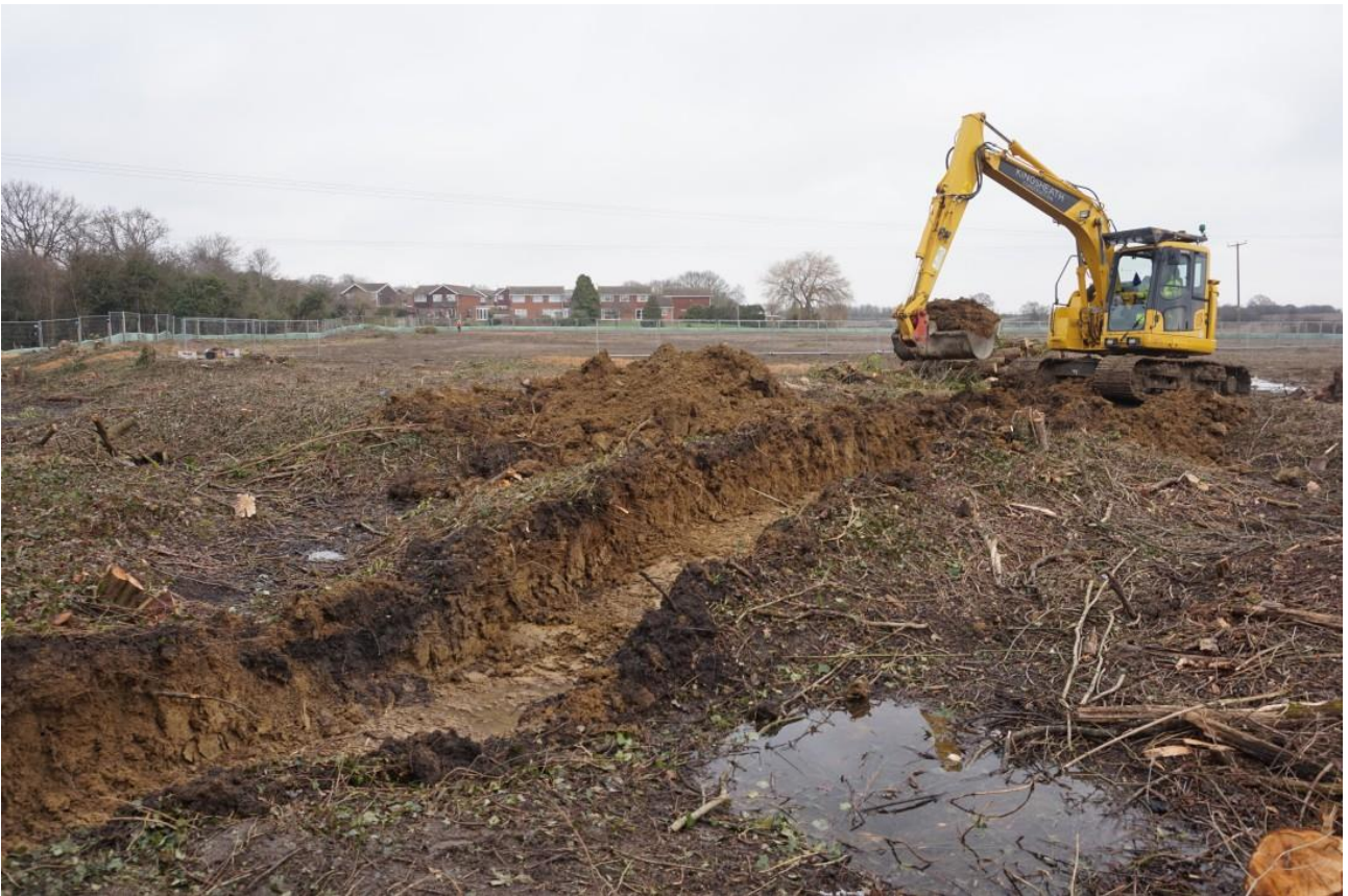
Plate 10. Trench 27 (looking N)
